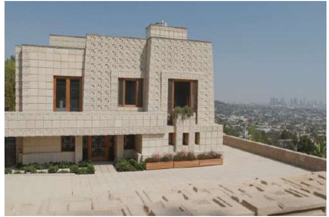
Concrete exterior, The Ennis House (1924)
