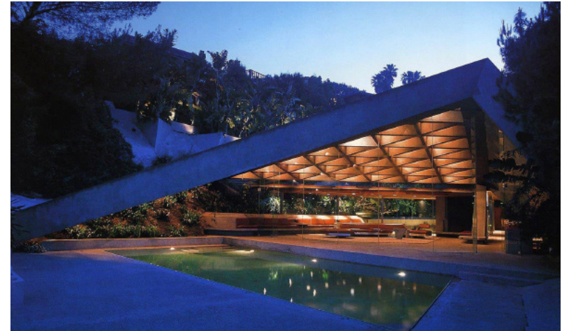
John Lautner, Sheats-Goldstein House, Los Angeles, CA, 1961-1963
